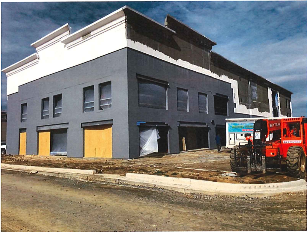
Side view under construction from Robins Way SW
